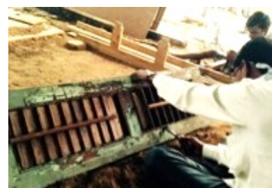
Figure 3. Local carpenters restoring old wooden door for a residential project. (Photo Credit: Artha Studio)
